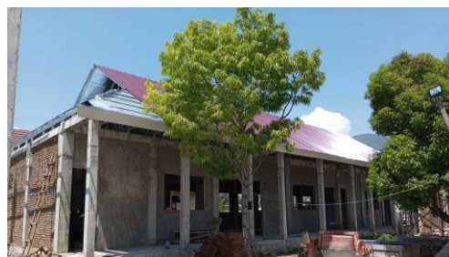
The reconstruction of classroom in SDN Pengawu in Palu City.
