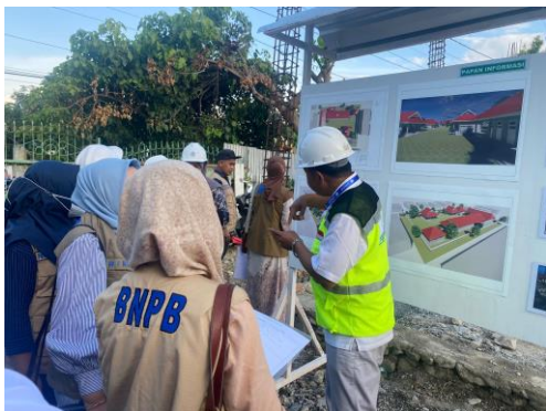
Joint monitoring to the school reconstruction in SDN Pengawu.
